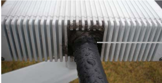
Weatherproof sealant applied to conduit cable connection to the Sharp.
